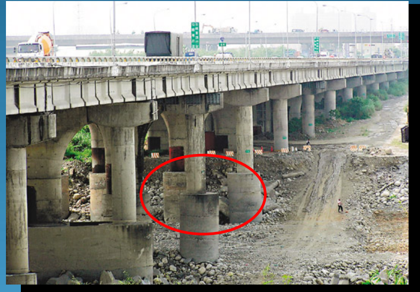
High scouring depths after many flood's phenomena
